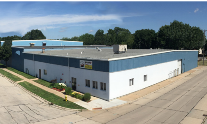
40,000 SF Facility - 24,000+ SF Under Crane
